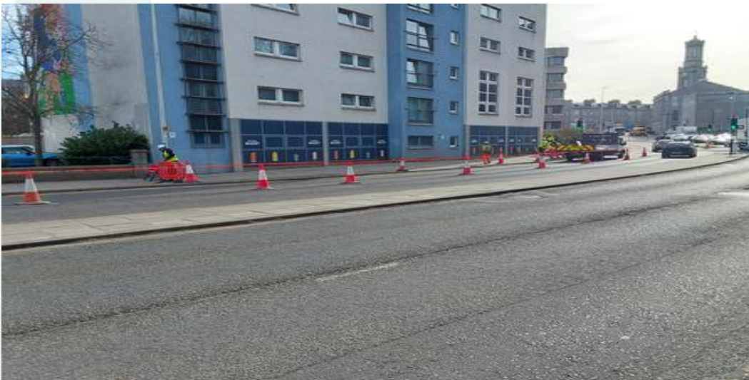
Phase 4 scaffolding lane closure and footpath restrictions.
